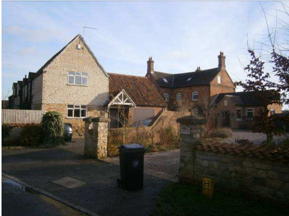
View of original structures from 19 th century either converted or extended and used as dwellings. Building on left has been extended to include a new first floor.
