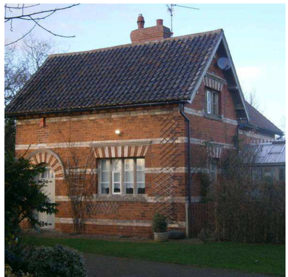
Photo shows Nightingale Cottage with elaborate Victorian detailing to window heads, stone mullions and banded brickwork.
