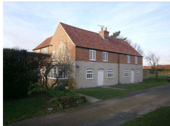
Former cottages converted into one single dwelling with evidence of extensions both to the rear and upwards to create a first floor. The side walls incorporate the original stone gable.
