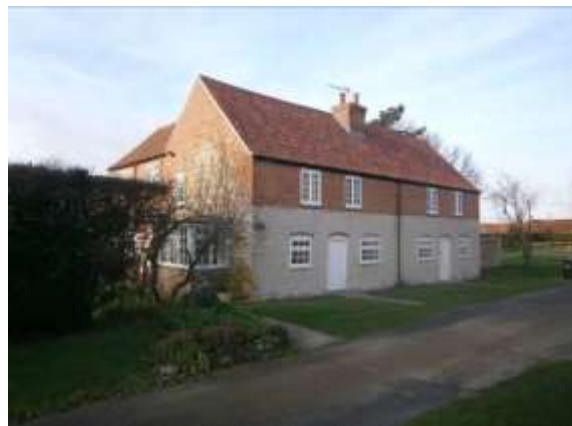
Former cottages converted into one single dwelling with evidence of extensions both to the rear and upwards to create a first floor. The side walls incorporate the original stone gable.
